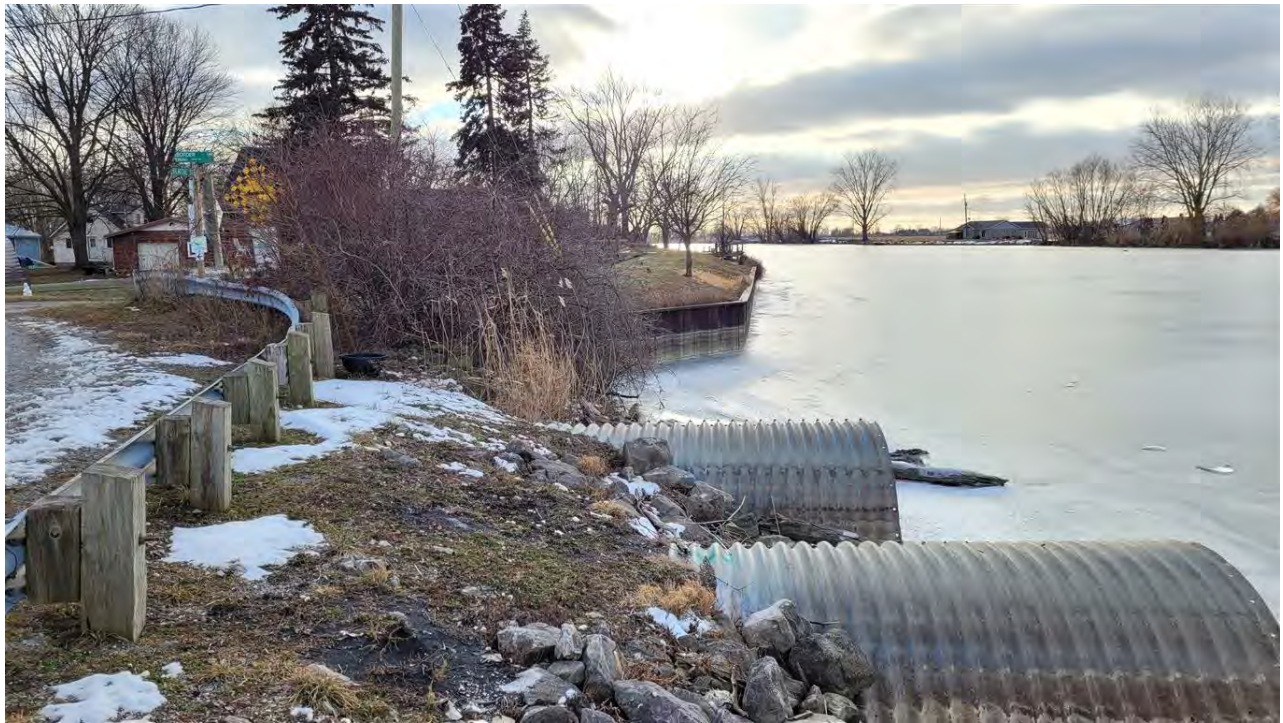
Image 31: Previous disturbance of the Sydenham River bank within the ROW of Border Road; sheet piling, bank stabilization, and culverts; facing southwest, January 14, 2022 (Map 10H).
