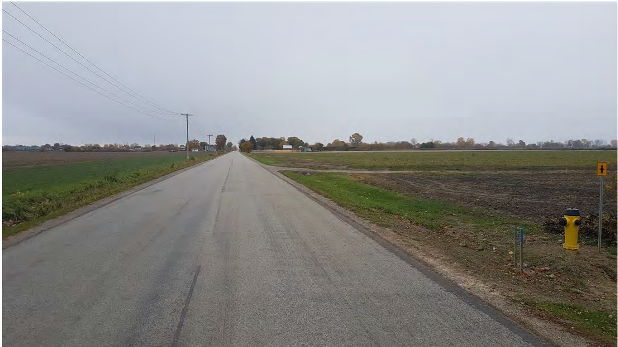
Image 16: A representative example of previous disturbance within the ROW of Base Line between the Potential New LLPS and WTP Areas; road, road embankments, drainage ditches, and buried utilities; facing east, October 27, 2020 (Map 10D).
