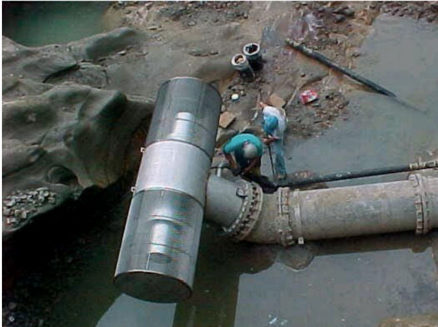
Figure 5-3. Submerged Tee Screen Installation (Courtesy of Johnson Screens)
