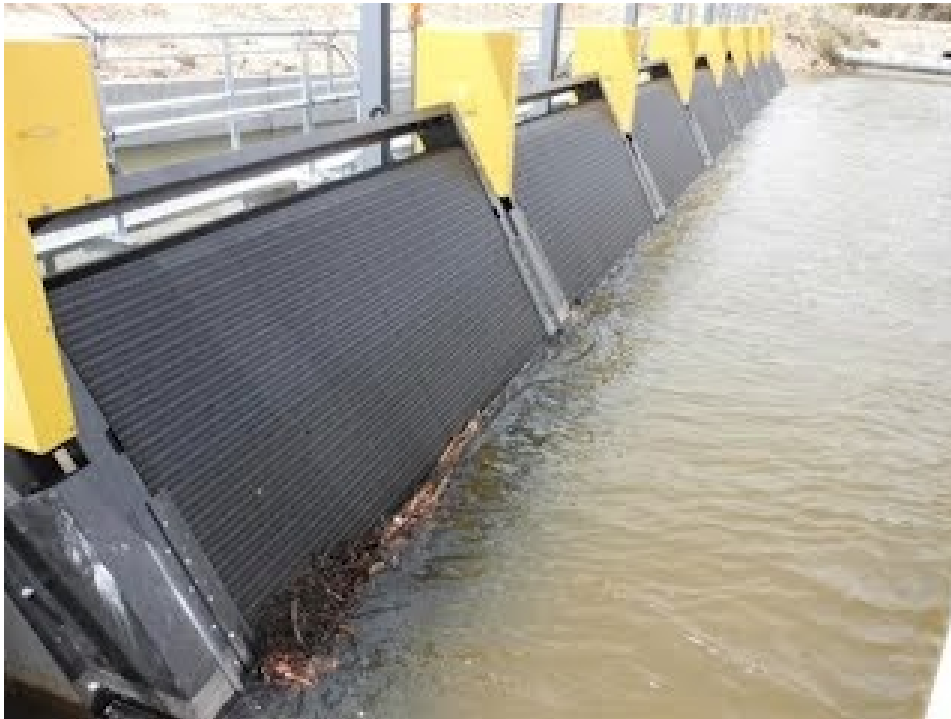
Figure 5-7. Flat Panel Fish Screens (Courtesy of OneFish Engineering)
