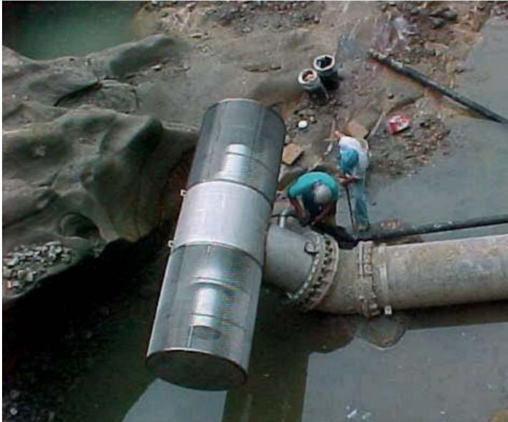
Figure 8-4. Example Installation for Intake Screens
