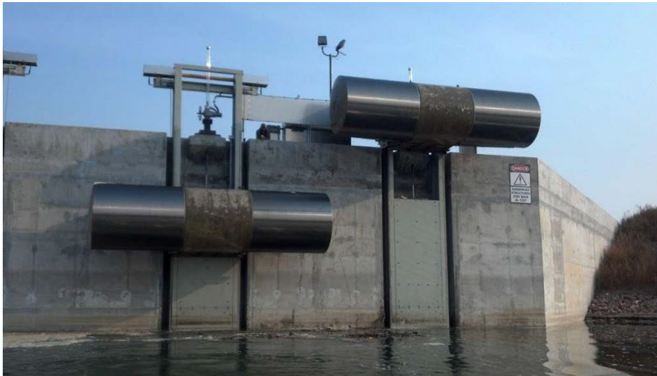
Figure 5-5. Headwall-Mounted Tee Screens (Courtesy of ISI Screens)
