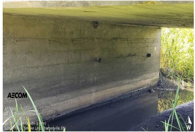
Photograph 30. ↑ Barn swallow nest under bridge. Water Crossing 1237-11651 on Smoke Line
