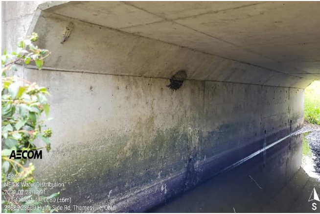
Photograph 29. ↑ Barn swallow nest under bridge. Water Crossing 23686 23600 on Huffs Side Road
