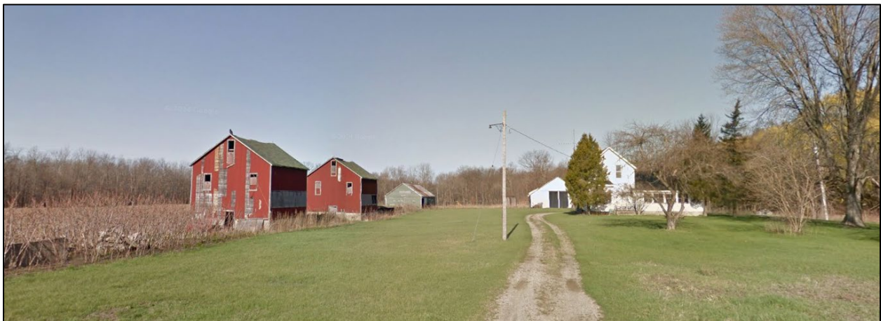
Looking west towards the existing dwelling and outbuildings on the severed parcel described as Part 2 on the applicant's sketch, from Clachan Road.
