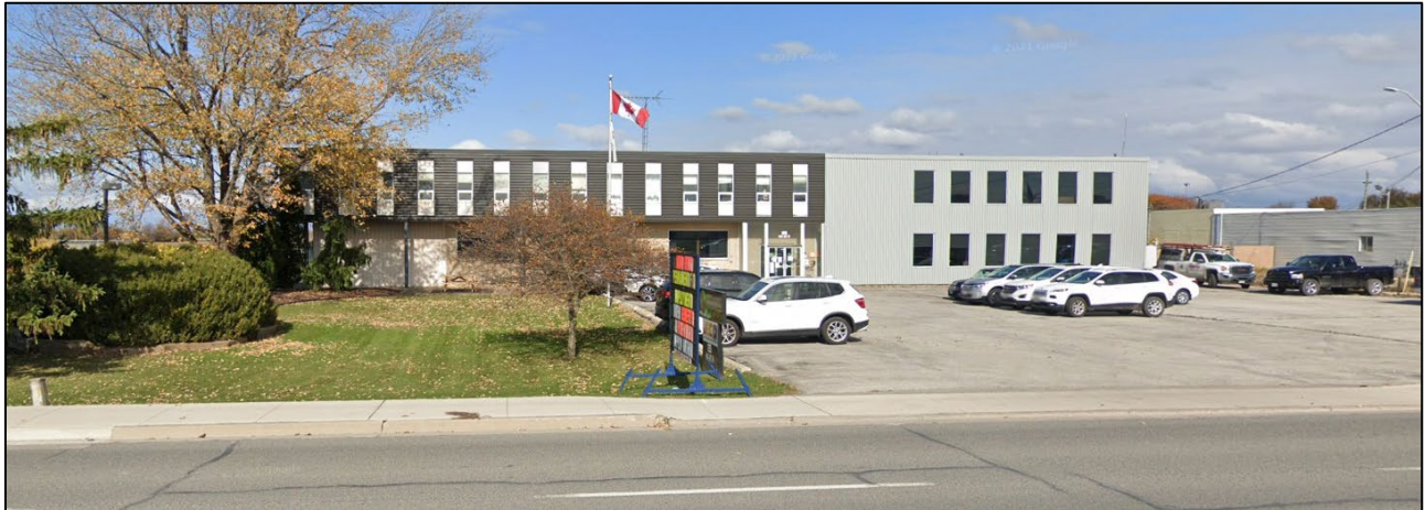
Looking north towards the existing industrial building on the proposed retained parcel, from Mill Street West.
