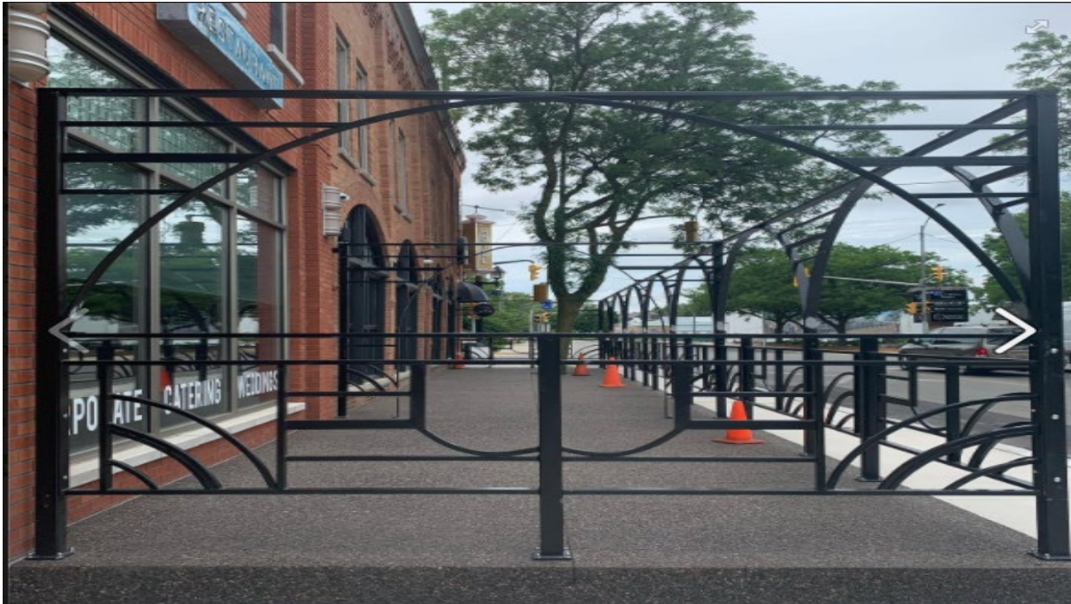
Looking north at the new patio.
