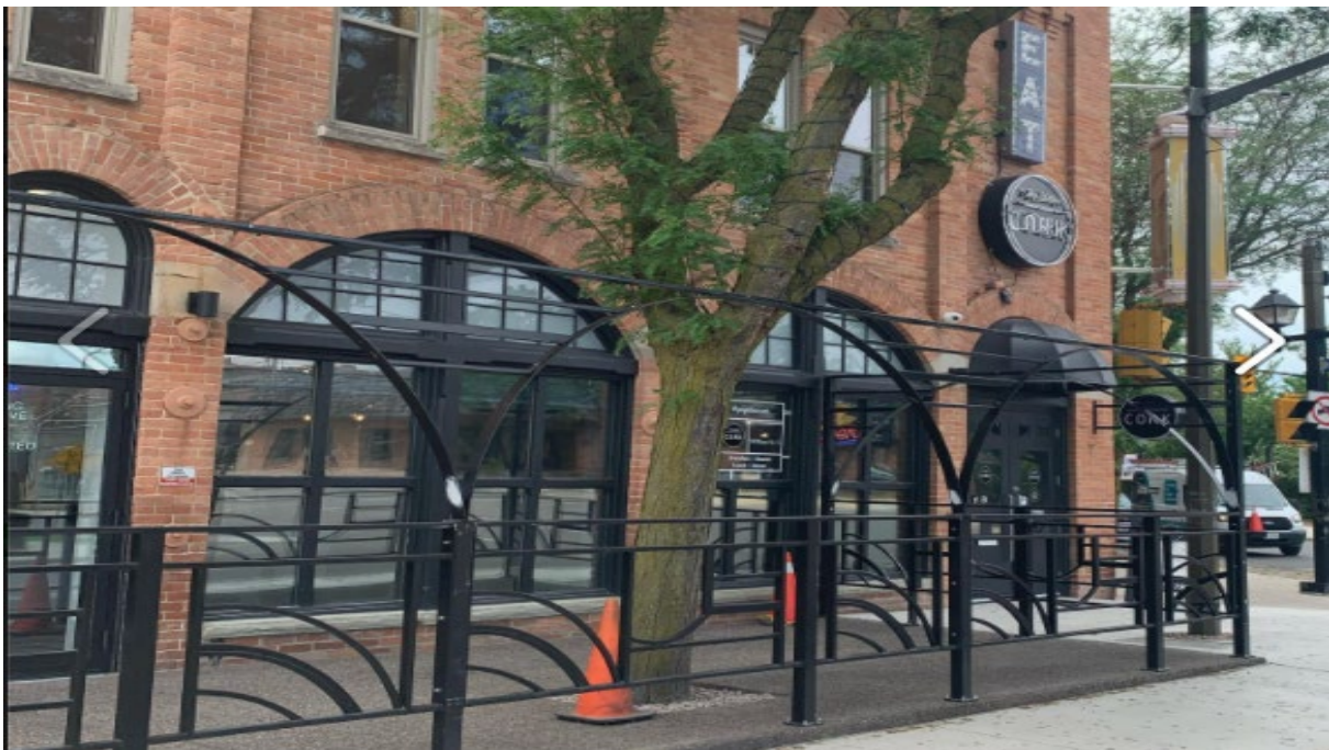
Looking west at the new patio.
