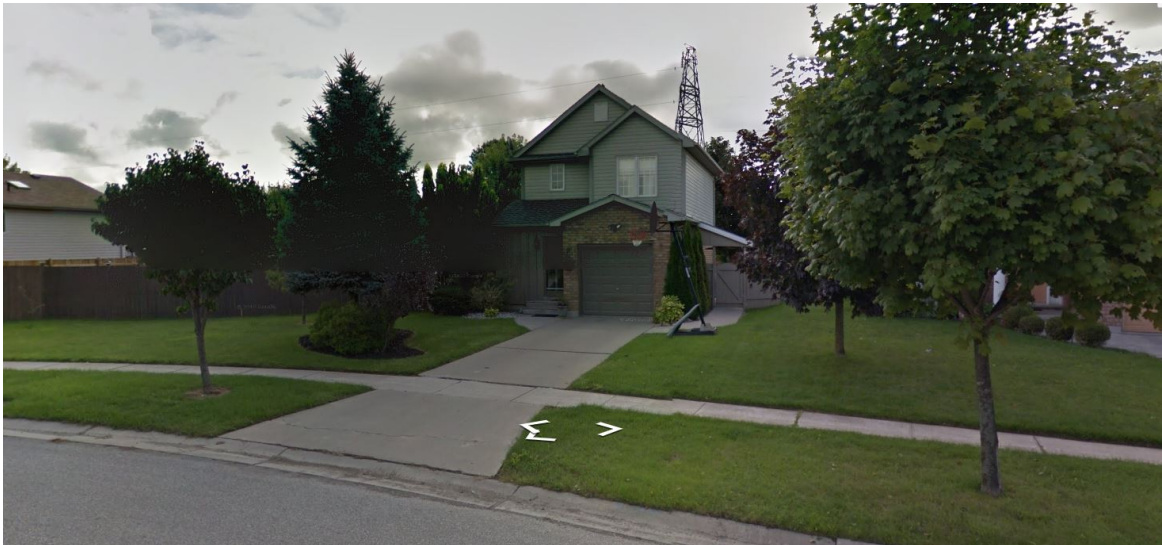
Looking south across the subject lands from Bristol Drive. In view is the existing dwelling on the subject lands.
