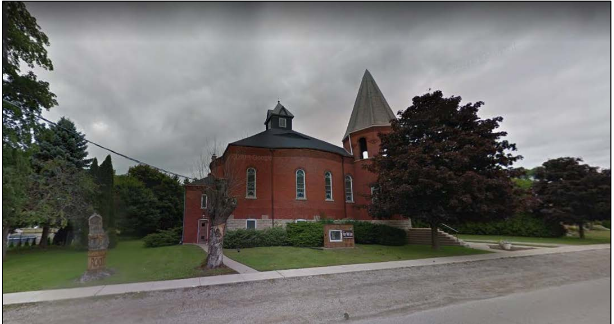
Looking north at the Mary Webb Cultural and Community Centre on the retained parcel.
