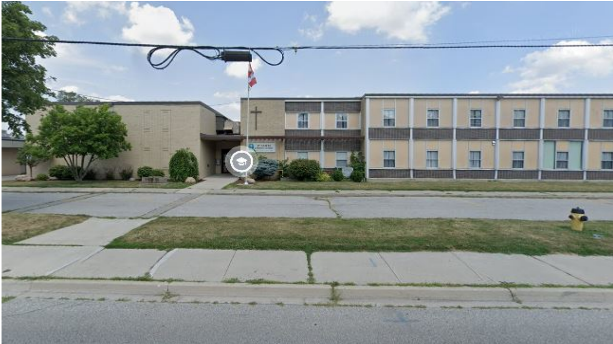
Looking northeast at the existing building on the property.
