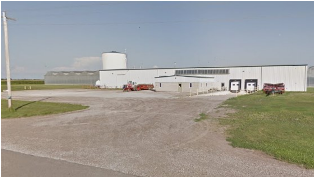
Looking east at the existing service building from Rivard Line.
