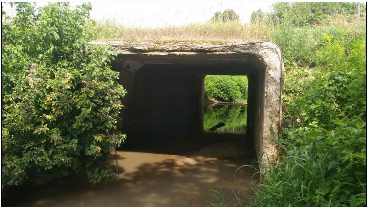
Figure 1. New Scotland Line over Ross Drain – South Culvert End
