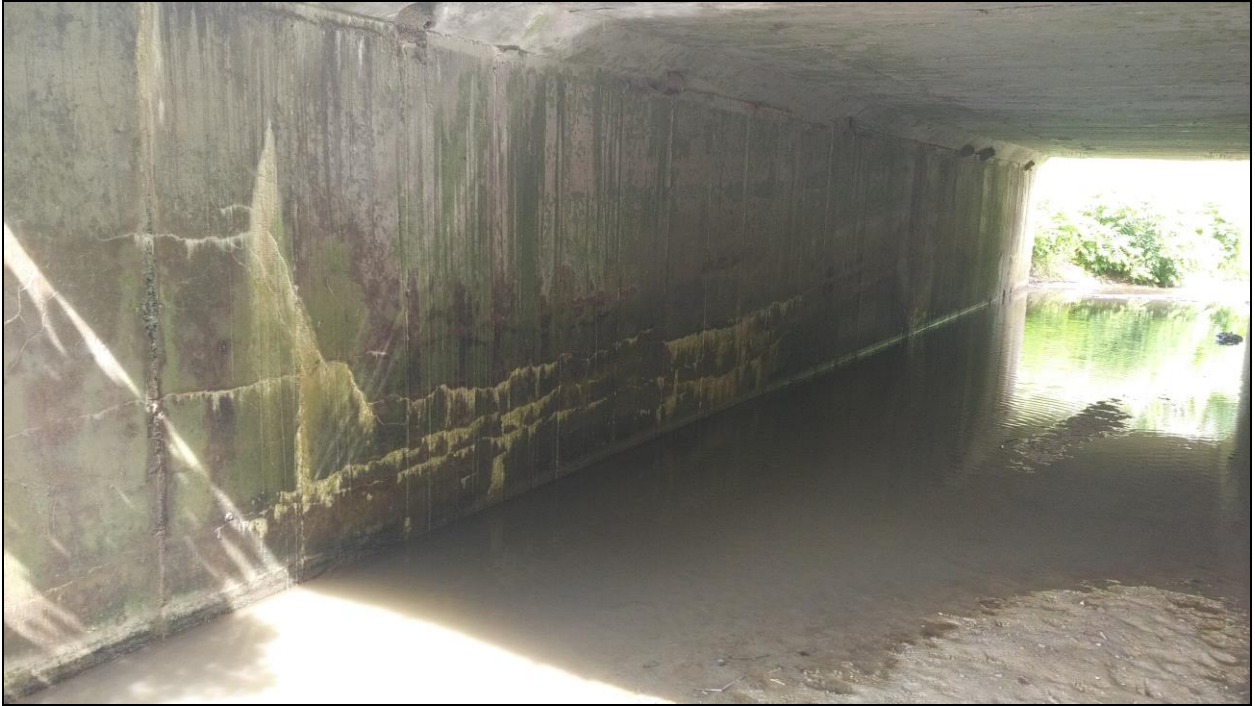
Figure 2. New Scotland Line over Ross Drain – Interior Barrel
