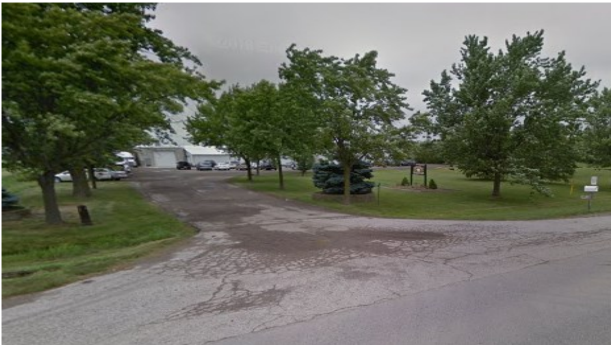
Looking north at the existing facility across Middle Line.
