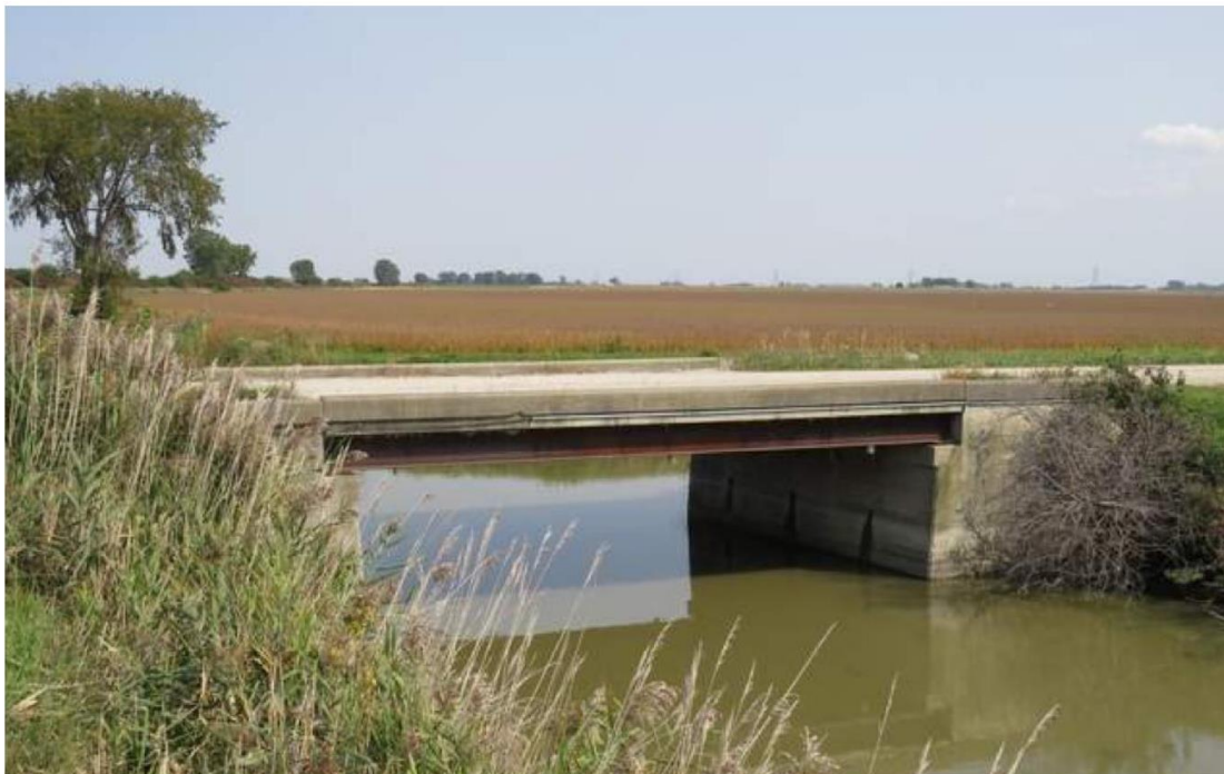
Figure 1. Dauphin Road Bridge over Dauphin Internal Drain
