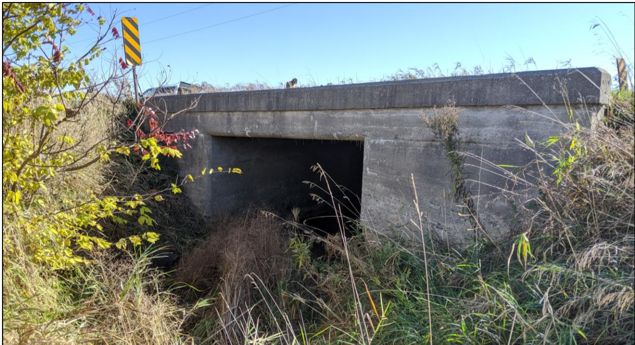
Figure 1. McKay's Line over Fields Creek Drain – Northwest Culvert End
