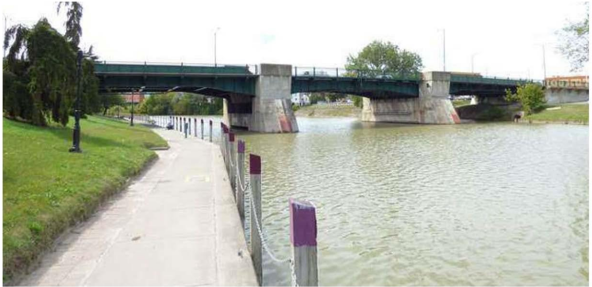
Figure 1. Photo of the existing Third Street Bridge over the Thames River
