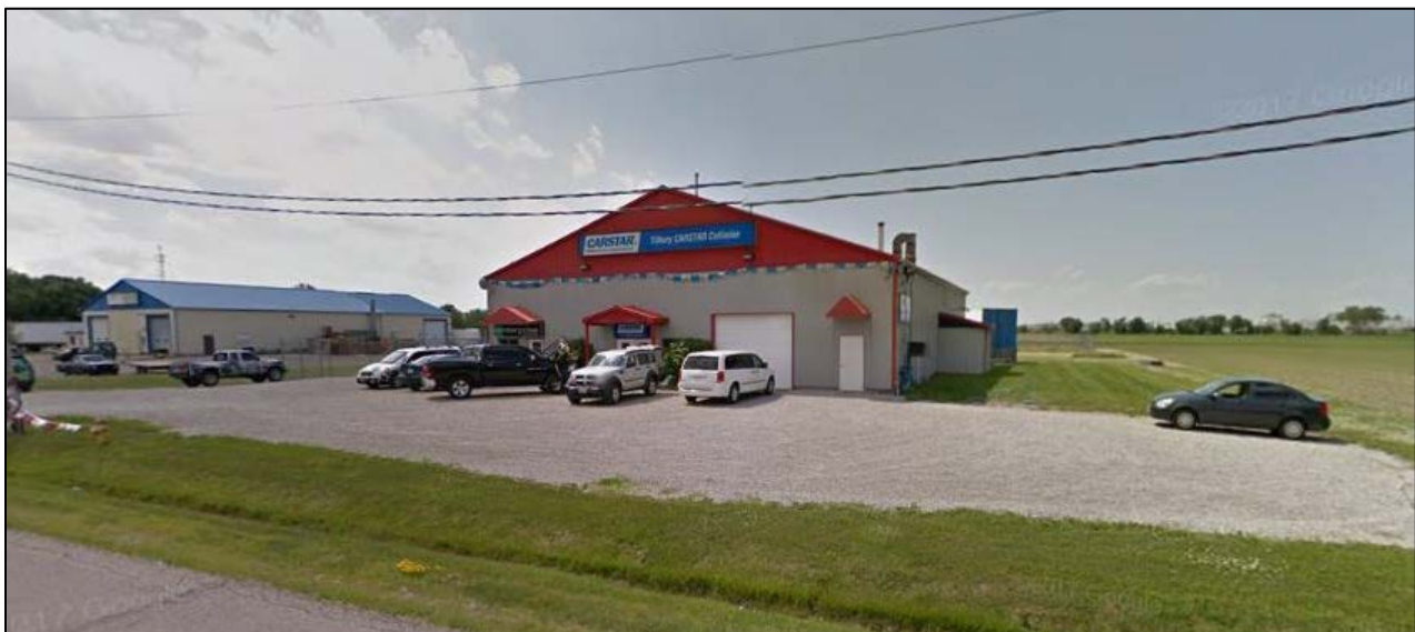
Looking northwest at the subject property from Wheeler Line.
