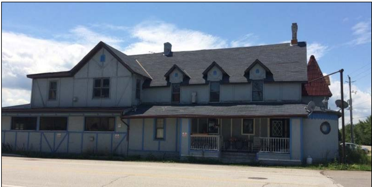
View of existing building from Winter Line Road.
