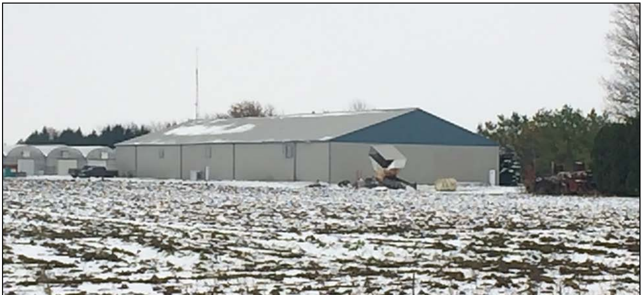
The existing enclosed accessory building to contain the commercial cannabis operation.
