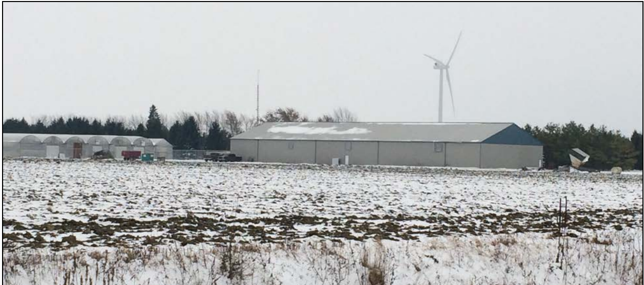
Looking south across the subject property from Mallard Line. The existing enclosed accessory building to contain the commercial cannabis operation and the existing greenhouses to the left.
