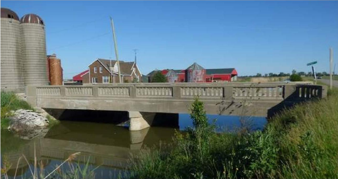
Figure 2. Overall view of the McDougall Line Bridge over Government Drain #1
