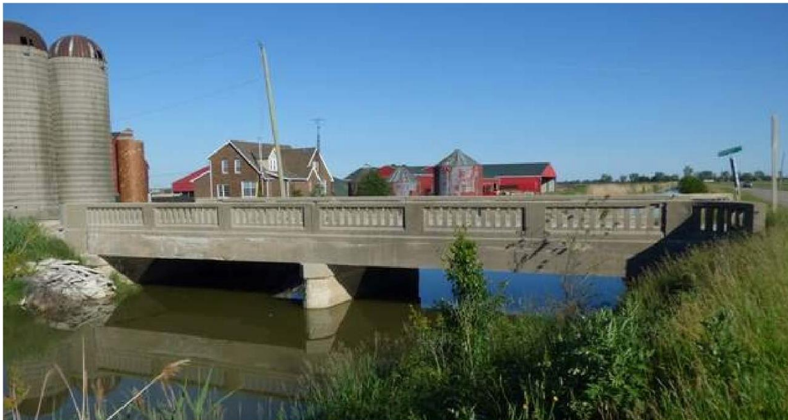
Figure 1. McDougall Line Bridge over Government Drain #1
