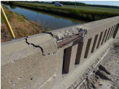
Figure 3. Underside view of deck and girders and top view of concrete railing
