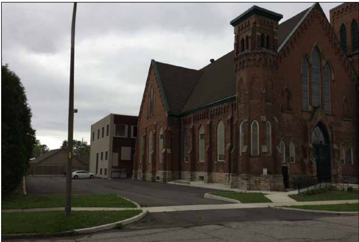
Looking west across the subject property from Dufferin Avenue.
