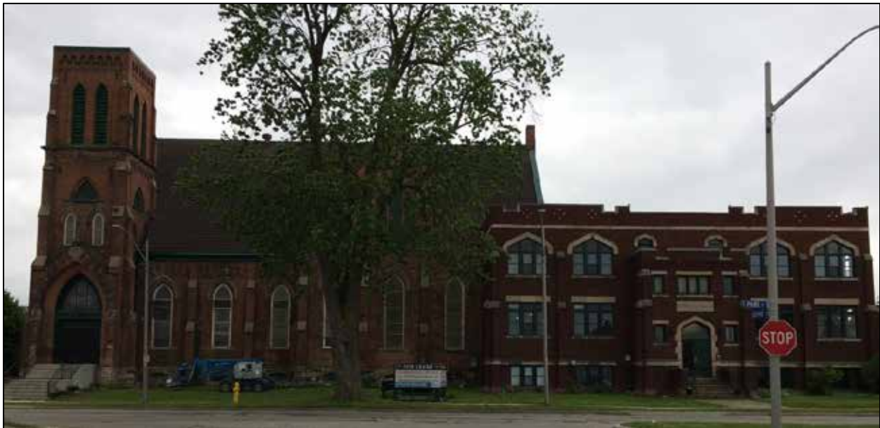
Looking south across the subject property from Park Street.
