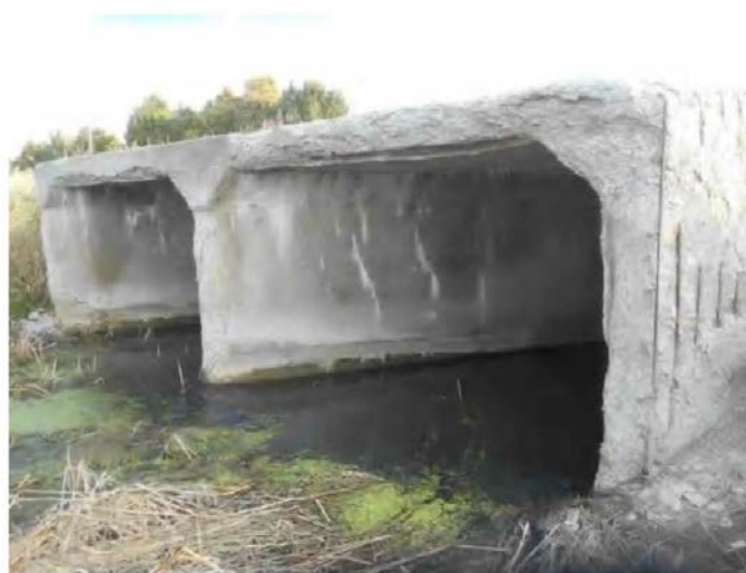
Figure 1. Lindsay Road over Big Creek
