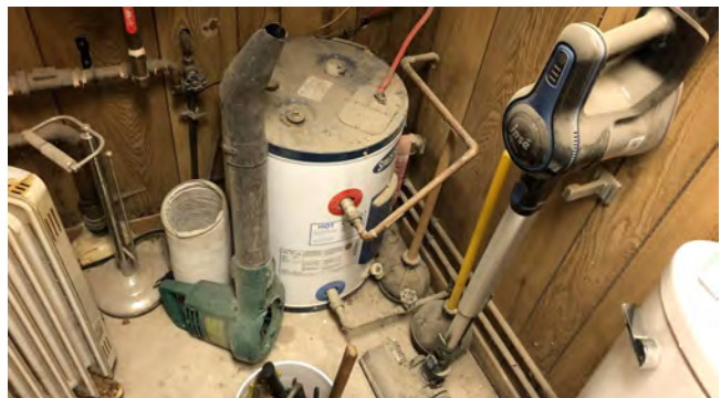
Replacement of domestic hot water heater required at Dover waste depot
