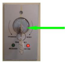
The magnetic locks must be manually reset after a power failure. Following the power failure the green light should be lit up indicating the doors are released. To secure them turn the key to the right and then back to the centre position. When the doors are secure the red light should be on, as shown in this diagram.
