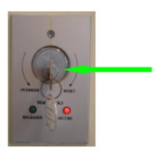
The magnetic locks must be manually reset after a power failure. Following the power failure the green light should be lit up indicating the doors are released. To secure them turn the key to the right and then back to the centre position. When the doors are secure the red light should be on, as shown in this diagram.
