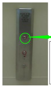
On both elevators, turn the key in the fire recall slot, as shown in the pictures, on the elevator panel to "reset" and then back to the neutral position.
