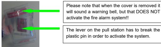
ii. Activate the pull station by pulling the lever towards you. Before walking away from the pull station ensure the fire system activates. If it doesn't sound the alarm and lights make sure you have pulled the lever all the way. If the system still does not activate proceed to another pull station and notify the Incident Manager of the issue so it can be included on the Fire Alarm Report.
