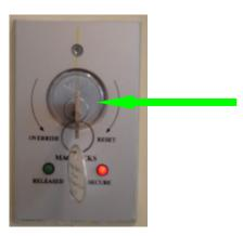
The magnetic locks must be manually reset after a fire alarm. Following a fire alarm the green light should be lit up indicating the doors are released (i.e. unlocked). To secure the door turn the key to the left to turn off the green light and then to the right all the way to secure the doors and then back to the centre position. When the doors are secure the red light should be on, as shown in this diagram.
