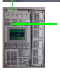
To reset the panel push the button under the RESET button.
