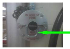
The fire suppression system in the main kitchen is automated and should not be used manually unless there is a significant fire with the potential of spreading.
