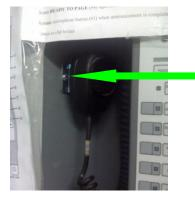
To operate the microphone hold down the button on the side of the microphone. (It will take a few seconds for the microphone to be operational). Hold the microphone 8 - 10 inches from your mouth and speak clearly and slowly. When you are done speaking release the button on the side. (Any time the button is held down the microphone is operational and the entire building can hear what you are saying!)
