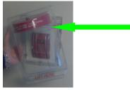
This is the plastic cover that needs to be removed in order to access the pull station. Please note that when the cover is removed it will sound an alarm, it is not connected to the fire system. You must still pull the lever on the pull station.
