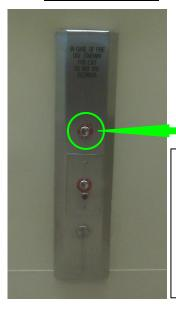
On both elevators, turn the key in the fire recall slot, as shown in the pictures, on the elevator panel to "reset" and then back to the "off position.
