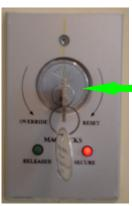
The magnetic locks must be manually reset after a fire alarm. Following a fire alarm the green light should be lit up indicating the doors are released (i.e. unlocked). To secure the door turn the key to the left to turn off the green light and then to the right all the way to secure the doors and then back to the centre position. When the doors are secure the red light should be on, as shown in this diagram.
