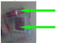
Please note that when the cover is removed it will sound a warning bell, but that DOES NOT activate the fire alarm system!!
