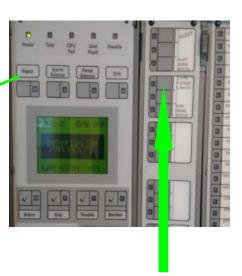
To stop the system from going into a Fire Alarm Signal press the "Evac Timer Cancel" button on the enunciator panel.
