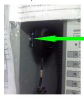
To operate the microphone hold down the button on the side of the microphone. (It will take a few seconds for the microphone to be operational). Hold the microphone 8 – 10 inches from your mouth and speak clearly and slowly. When you are done speaking release the button on the side. (Any time the button is held down the microphone is operational and the entire building can hear what you are saying!)
