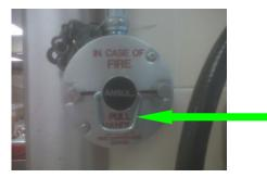
The fire suppression system in the main kitchen is automated and should not be used manually unless there is a significant fire with the potential of spreading.
