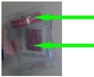
Please note that when the cover is removed it will sound a warning bell, but that DOES NOT activate the fire alarm system!!
