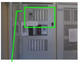
If the panel is indicating an ALARM, SUPURVISORY, TROUBLE or MONITORING condition, the issue that caused the system to signal an alert/alarm must be resolved before resetting the panel.
