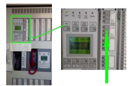
To stop the system from going into a Fire Alarm Signal press the "Evac Timer Cancel" button on the enunciator panel.
