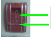
The Fire Alarm system is activated when the lever is pulled down breaking the plastic pin.
