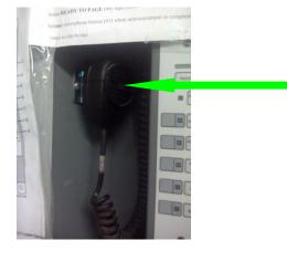
To operate the microphone press the button on the side hold, wait for the tone to stop, hold the microphone 8 - 10 inches from your mouth and speak clearly and slowly. When you are done speaking release the button on the side. (Any time the button is held down the microphone is operational and the entire building can hear what you are saying!)
