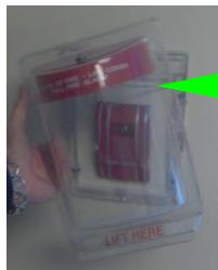
This is the plastic cover that needs to be removed in order to access the pull station. Please note that when the cover is removed it will sound an alarm, it is not connected to the fire system. You must still pull the lever on the pull station.
