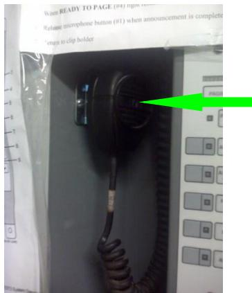
To operate the microphone press the button on the side hold, wait for the tone to stop, hold the microphone 8 – 10 inches from your mouth and speak clearly and slowly. When you are done speaking release the button on the side. (Any time the button is held down the microphone is operational and the entire building can hear what you are saying!)
