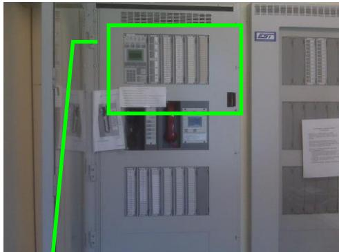
If the panel is indicating an ALARM, SUPERVISORY, TROUBLE or MONITORING condition, the issue that caused the system to signal an alert/alarm must be resolved before resetting the panel.
