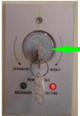
The magnetic locks must be manually reset after a fire alarm. Following a fire alarm the green light should be lit up indicating the doors are released (i.e. unlocked). To secure the door turn the key to the left to turn off the green light and then to the right all the way to secure the doors and then back to the centre position. When the doors are secure the red light should be on, as shown in this diagram.
