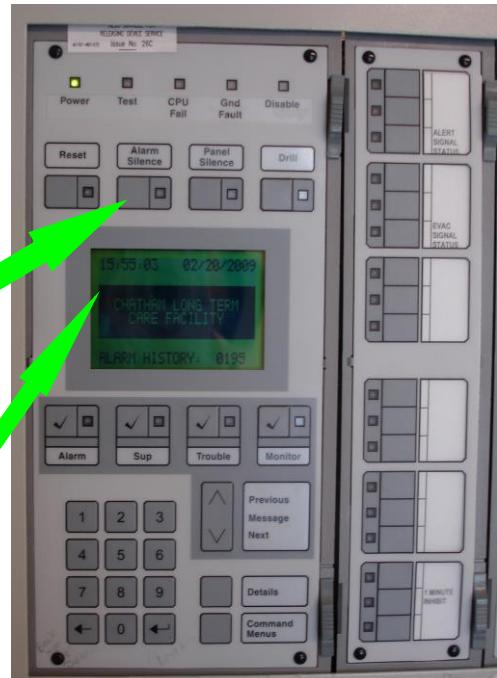
To silence the panel push the button marked Silent as shown here.
