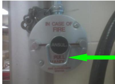
The fire suppression system in the main kitchen is automated and should not be used manually unless there is a significant fire with the potential of spreading.
