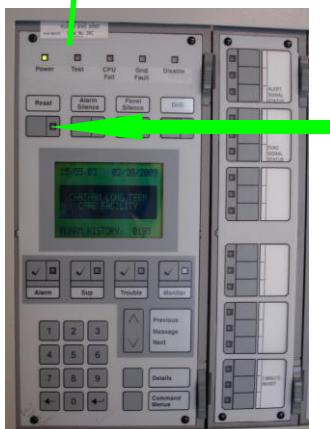
To reset the panel push the button under the RESET button.
