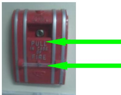
The Fire Alarm system is activated when the lever is pulled down breaking the plastic pin.
