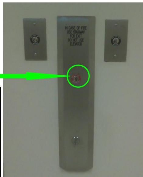
On both elevators, turn the key in the fire recall slot, as shown in the pictures, on the elevator panel to "reset" and then back to the "off" position.
