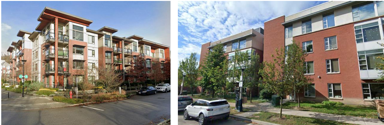
The images above demonstrate vertical articulations and colour blocking that are used to divide and soften the appearance of building massing. These design strategies can help medium and high density developments to fit within the context of lower density residential surroundings. Brick exteriors provide a heritage element that ties newer development in with older construction. (Images: Google Earth)
