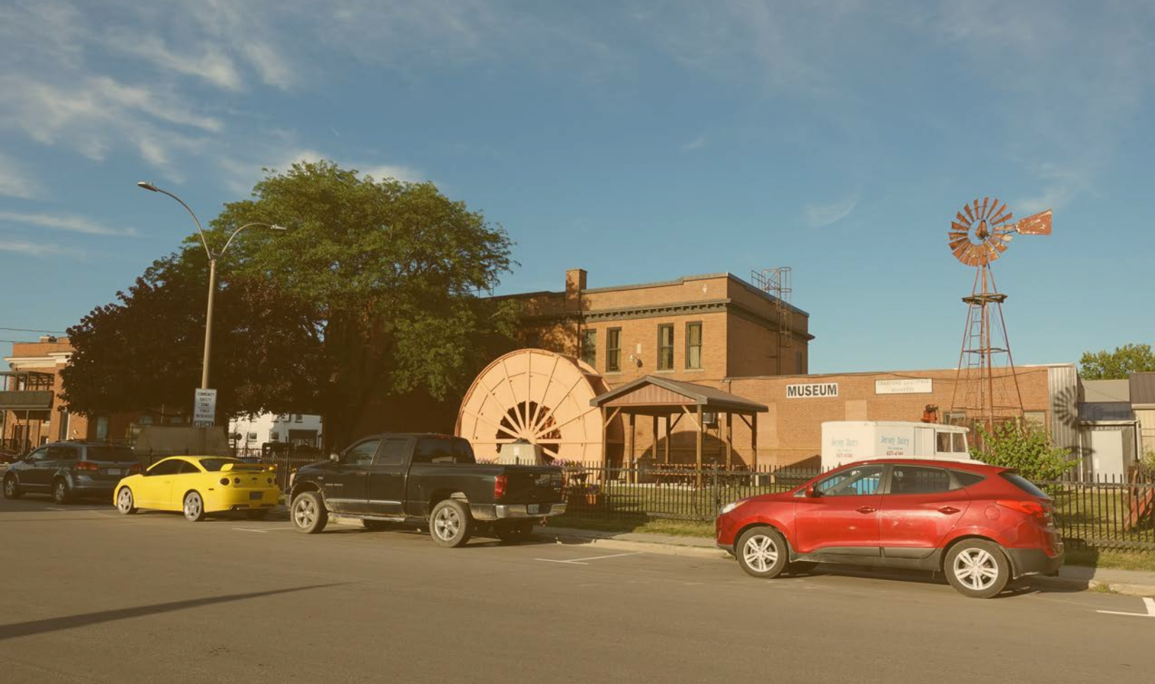
Above: Wallaceburg and District Museum and outdoor Agricultural Exhibit on King Street (view from Herbert Street).
