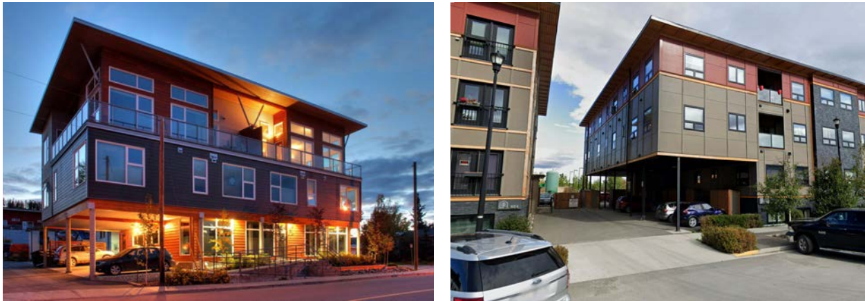
Carport parking is encouraged to increase the development potential of high density properties while softening the presence of parking next to the waterfront and providing opportunities for sheltered parking. The above image on the left shows a development with a commercial first storey and residential apartments on upper floors (Image: Kobayashi+Zedda Architects). On the right is a residential development (Image: Google Earth).
