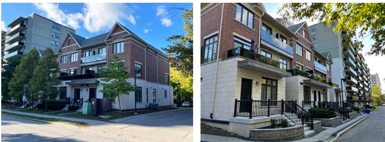
The above images show front and rear views of a back-to-back townhouse development with third storey apartments accessed through separated first storey entrances. The rear of the building is accessed from an internal drive with street-like treatment, including a sidewalk and curb.
