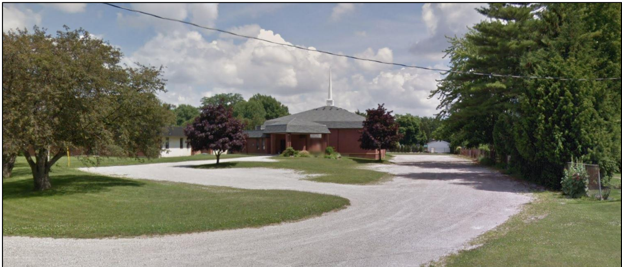
View of the subject lands from Crerar Drive. Picture depicts existing gravel area to the rear of the existing structure.
