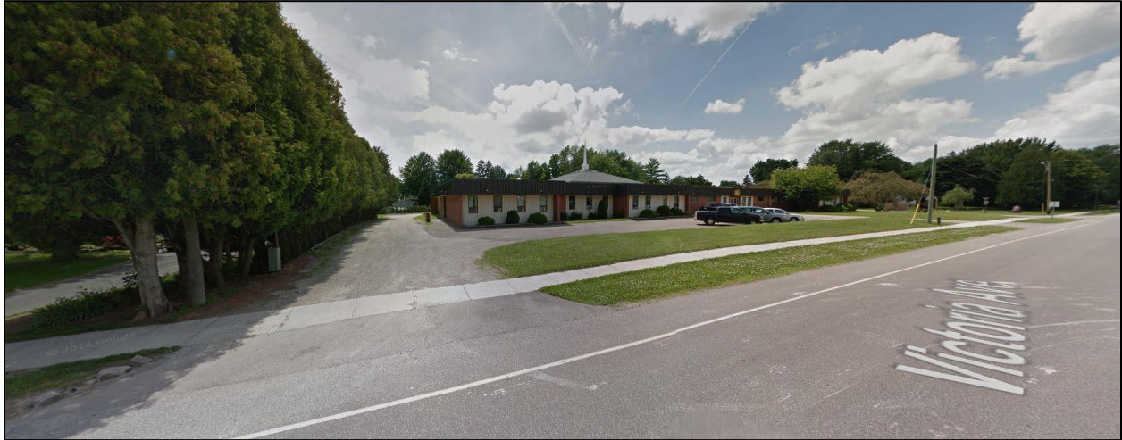
View of the subject lands and the most southerly entrance from Victoria Avenue.
