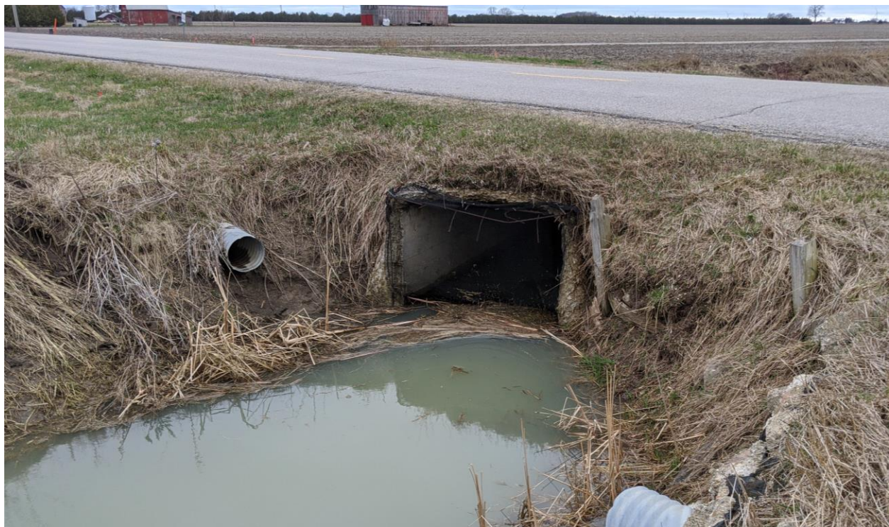
Figure 1. Union Line over Pollock Drain – South Culvert End
