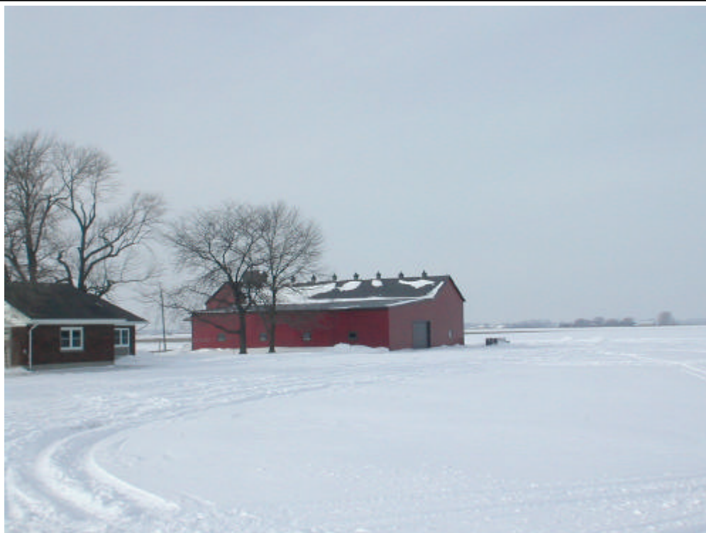
Looking northwest at the outbuilding to remain with the retained lands being conveyed to the abutting farm lot
